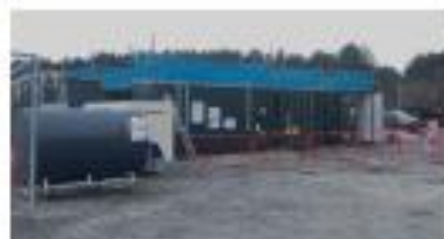
Pilot Plant components on site
